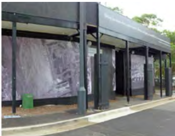
Example 13: Gantry Style – Acceptable in all zones
