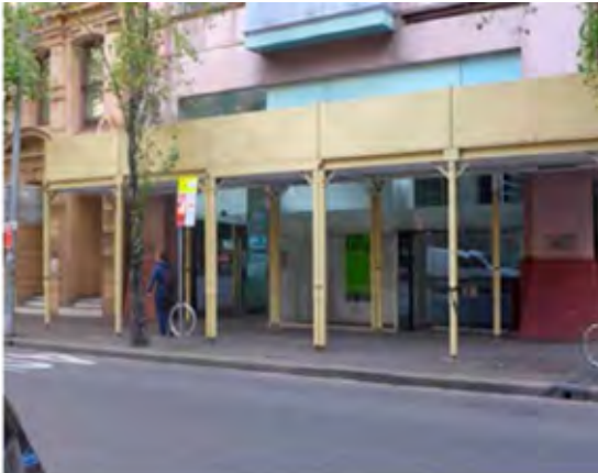
Example 11: Gantry Style – Acceptable in all zones
