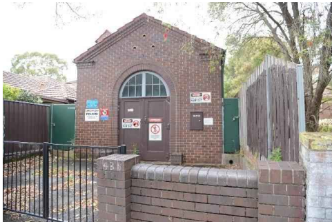
Figure 6.3 Heritage listed substation at 2B Cooper Street.
