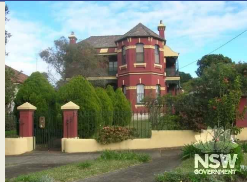
Figure 7.22 23 Badminton Street, Croydon, within its garden setting, July 2020 (Source: NSW SHI)
