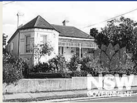
Figure 7.4 Primary elevation of 12 Belgrave Street, Burwood, July 1986. (Source: NSW SHI)
