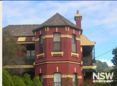
Figure 7.21 Primary elevation of 23 Badminton Street, Croydon, July 2020. (Source: NSW SHI)
