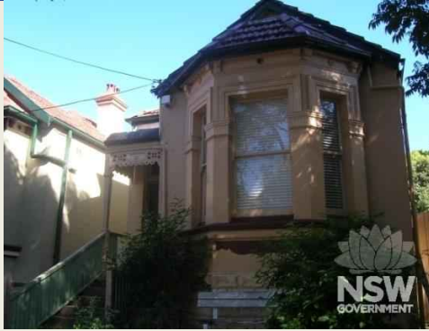
Figure 7.13 Primary elevation of 31 Wallace Street, Burwood, July 2020. (Source: NSW SHI)
