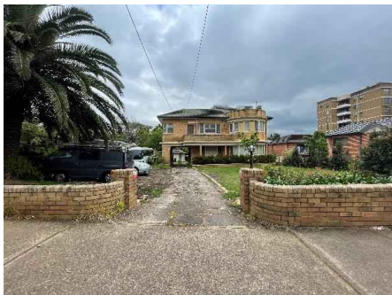
Figure 6.5 Heritage listed flats at 18A Cooper Street, Strathfield.
