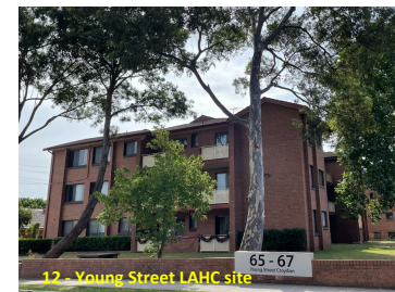
12 - Young Street LAHC site
