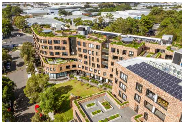
Arkadia, Alexandria. Medium density residential development with landscaped terraces and shared rooftop gardens. Source: Arch Daily
