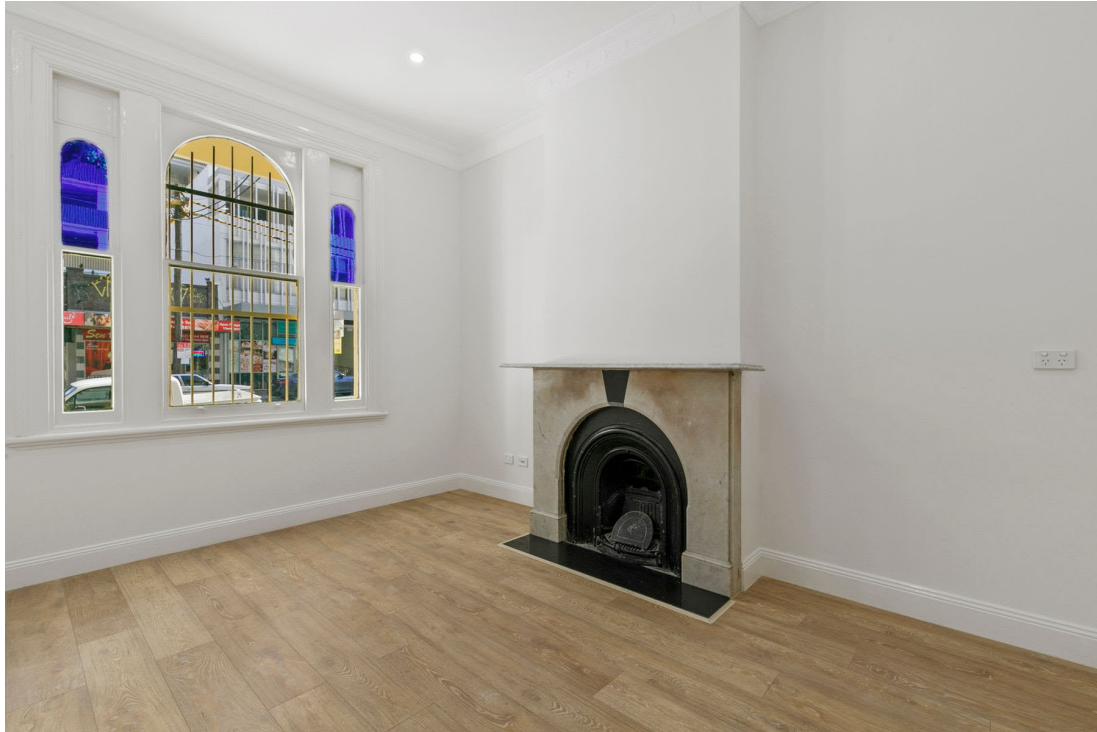
Figure 23 The ground floor of 12 Burwood Road c. 2021, showing intact fireplace and windows. (Source: RealCommercial.com.au)
