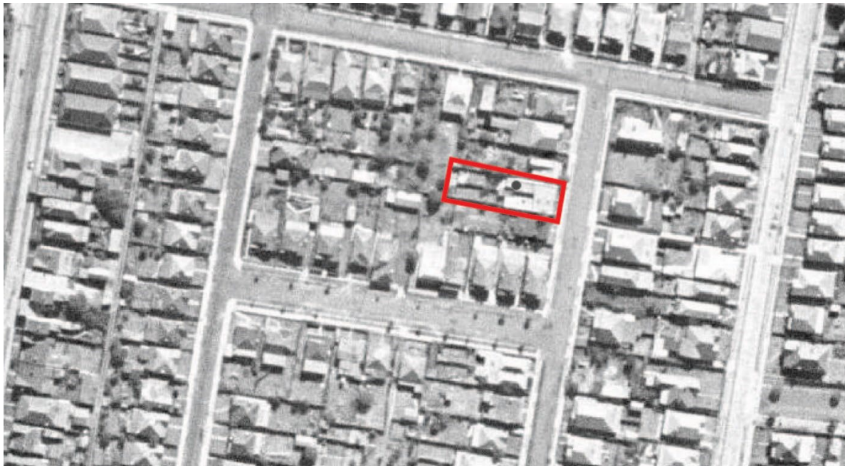
Figure 3 9-11 Archer Street, Burwood marked in red 1943. (Source NSW Historical Imagery, HAA overlay)
