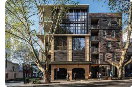
Figure 105: Small commercial tenancies with fine grain building articulation, Foveaux Commercial Suites. Source: Hill Thalys
