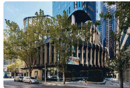
Figure 104: Articulated commercial & retail podium with tower over. Permeable public domain. Queen Place, VIC. Source: COX
