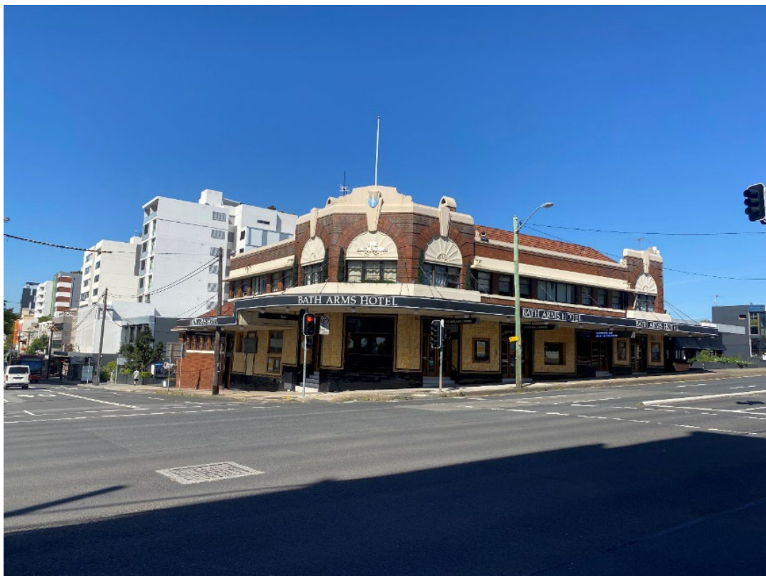
Figure 71 Bath Arms Hotel, 352-354 Parramatta Road, Burwood (Source: HAA)
