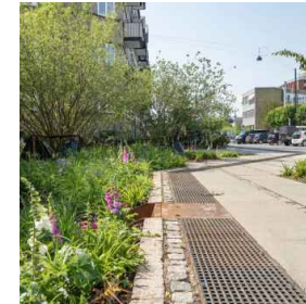
Figure 152: Storm water grate detail. Source: https://landezine-award.com/sankt-kjelds-square-and-bryggervangen/
