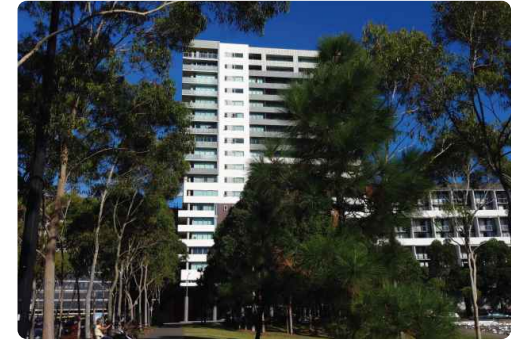
Figure 100: Residential medium-high density development opposite an open space. Victoria Park, Zetland. Source: COX
