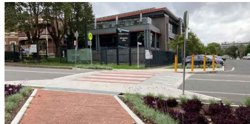
Figure 51: Traffic calming measure/ pedestrian cycle link. Source: COX
