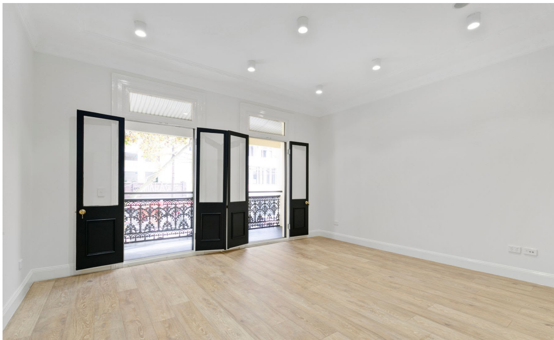
Figure 22 12 Burwood Road c. 2021, showing the upper floor with retained or reconstructed doors, architraves, balcony and skirting. Other features such as vents have been removed. (Source: RealCommerical.com.au)
