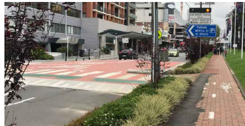
Figure 57: Raised threshold pedestrian/ cycle crossing - Burwood Road. Source: COX
