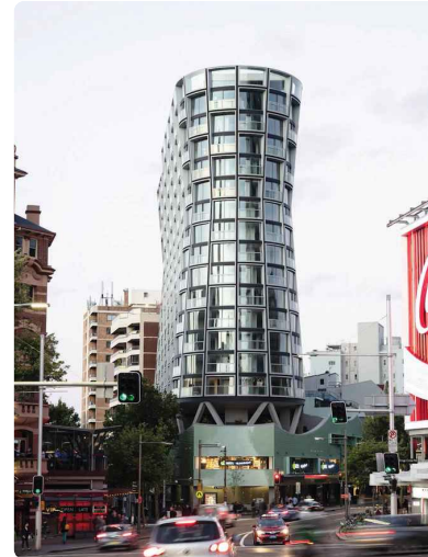
Figure 99: Mixed-use development with residential tower. Kings Cross, Durbach Block Jaggers. Source: COX
