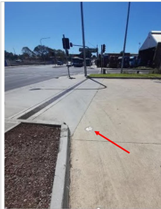
Photo 9: Monitoring well located within the footprint of 7-Eleven Petrol Station.
