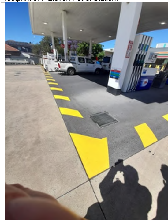
Photo 11: Bunded refuelling area around the bowsers on the 7-Eleven Petrol Station
