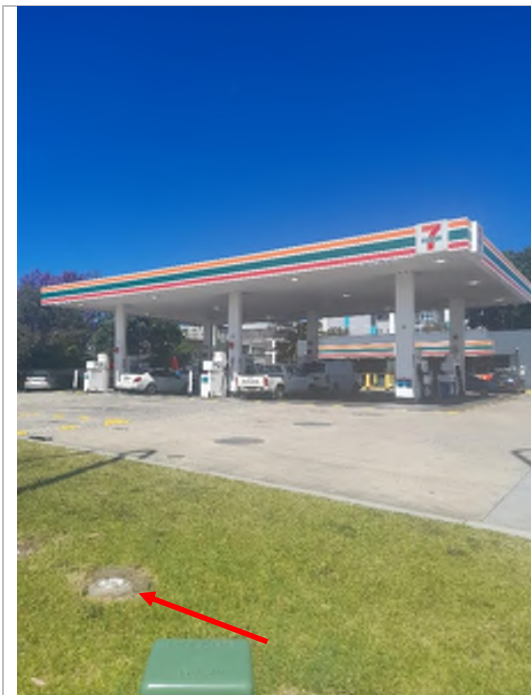
Photo 5: 7-Eleven petrol station showing concrete hard standing and a monitoring well (grassed area).
