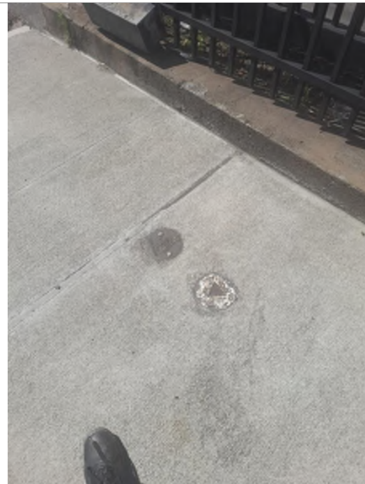
Photo 2: Monitoring well covers on the Parramatta Road pavement to the north of Burwood Bus Depot
