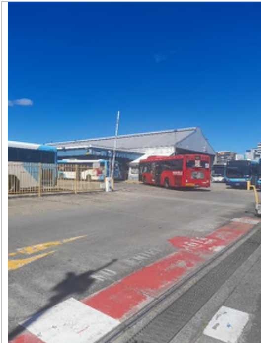
Photo 1: View from Parramatta Road looking south-west towards Burwood Bus Depot.
