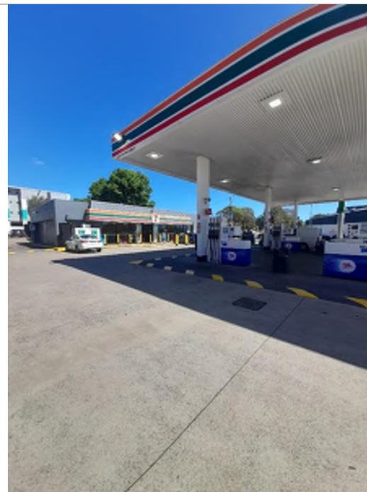
Photo 6: 7-Eleven Petrol Station showing concrete surfacing.
