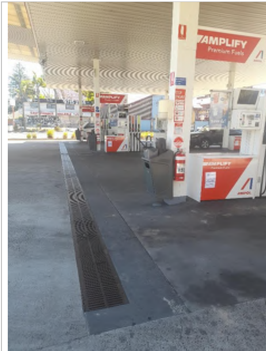
Photo 13: View of Ampol service station refuelling area.
