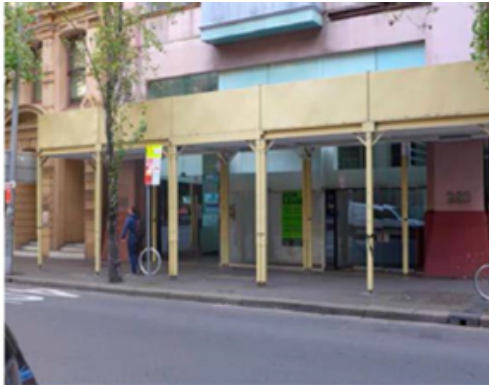
Example 11: Gantry Style – Acceptable in all zones
