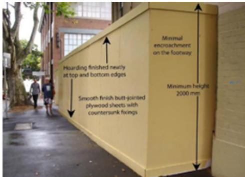
Example 5: Painted - Acceptable in Commercial Zones
