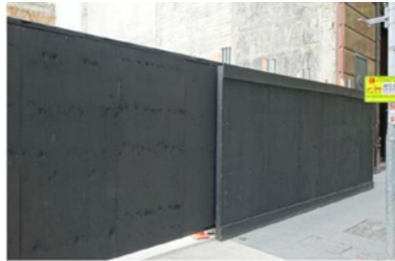
Example 6: Painted - Acceptable in Commercial Zones
