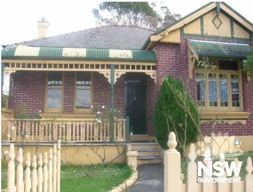
9 and 21 Seymour Street, Croydon Park
