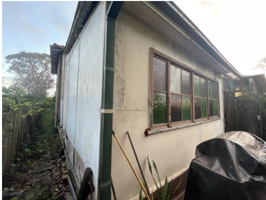
Figure 4.67 27 Woodside Avenue – kitchen addition
