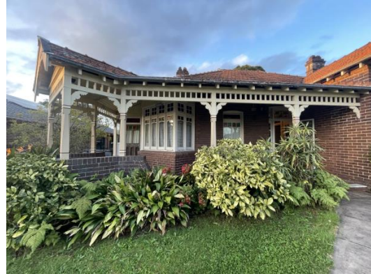
Figure 4.50 27 Woodside Avenue – front facade
