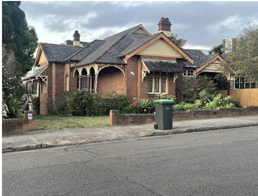
Figure 4.13 25 Woodside Avenue as seen from the street
