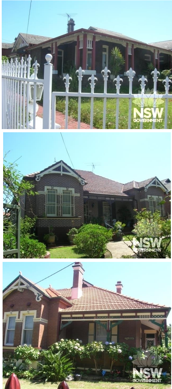
Figure 5.7 11, 17 and 19 Gladstone Street, Burwood (Source: NSW State Heritage Inventory)
