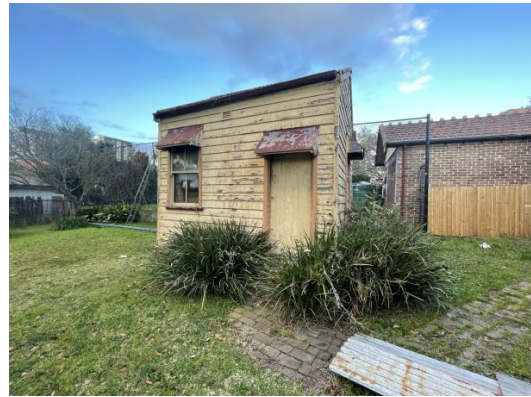
Figure 4.42 25 Woodside Avenue - outbuilding
