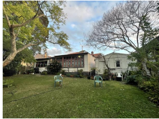
Figure 4.74 27 Woodside Avenue – rear of house and garage
