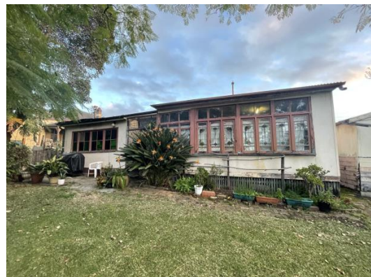
Figure 4.72 27 Woodside Avenue – rear of house
