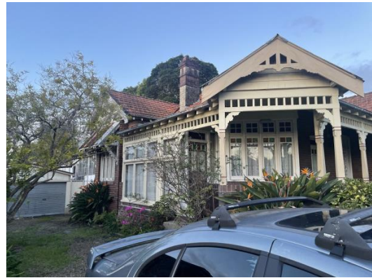
Figure 4.52 27 Woodside Avenue – corner detail
