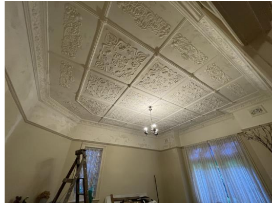
Figure 4.56 27 Woodside Avenue – ornate ceiling
