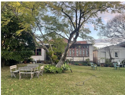
Figure 4.71 27 Woodside Avenue – rear of house
