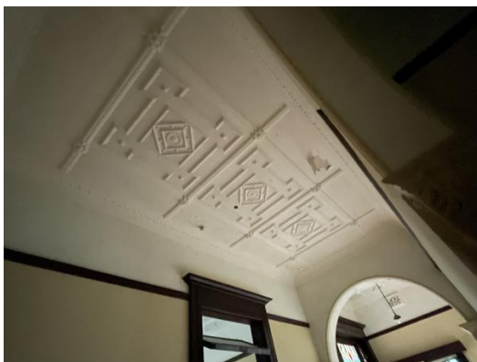
Figure 4.27 25 Woodside Avenue – ceiling detail
