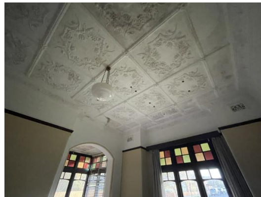
Figure 4.32 25 Woodside Avenue – ceiling detail
