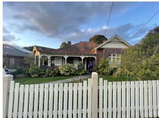
Figure 4.48 27 Woodside Avenue – front facade
