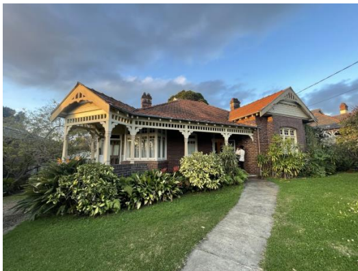
Figure 4.47 27 Woodside Avenue – front facade
