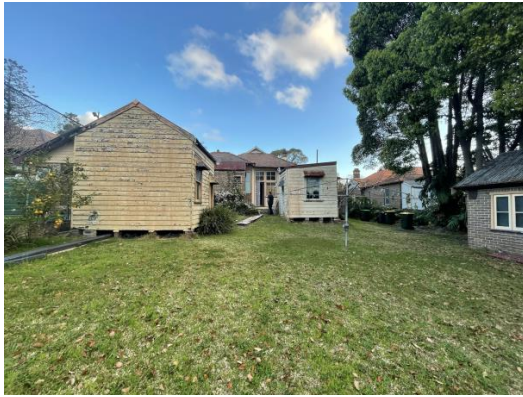
Figure 4.39 25 Woodside Avenue – rear of house
