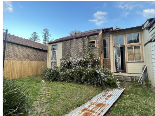
Figure 4.44 25 Woodside Avenue – rear of house
