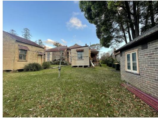
Figure 4.40 25 Woodside Avenue – rear of house
