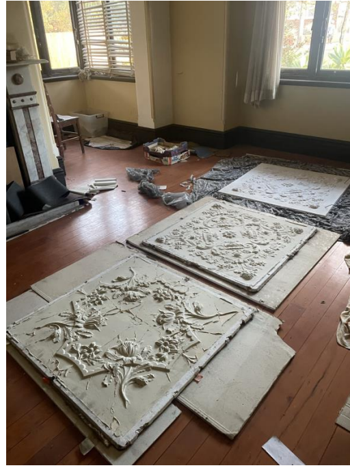
Figure 4.30 25 Woodside Avenue – ceiling repair detail
