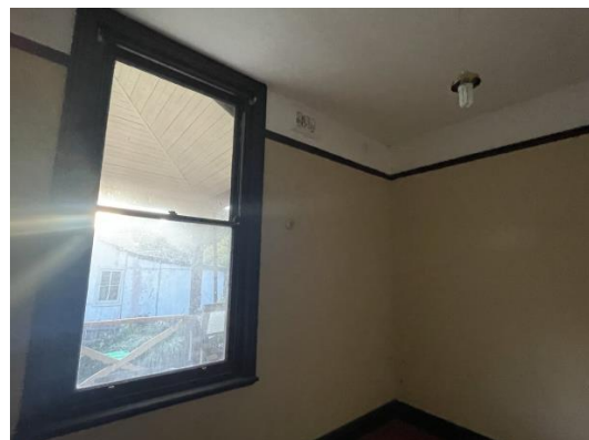
Figure 4.28 25 Woodside Avenue – bedroom window
