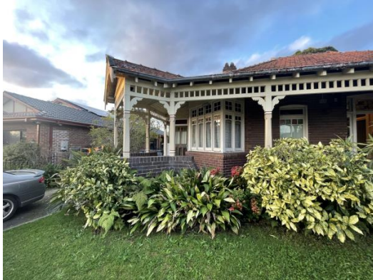
Figure 4.49 27 Woodside Avenue – front verandah
