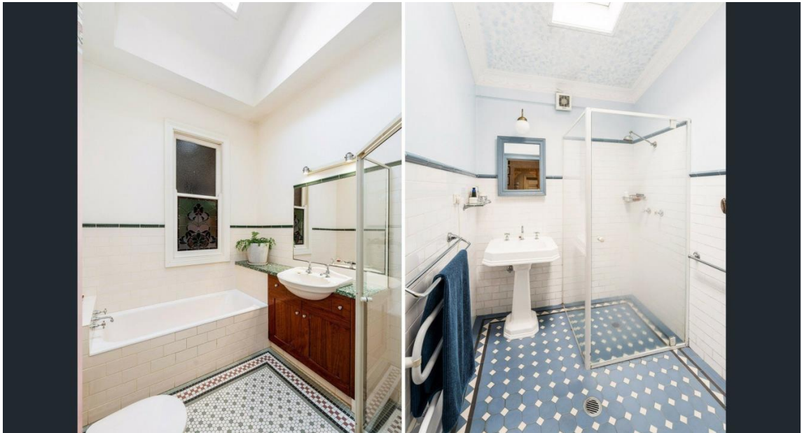
Figure 14 – View of altered bathrooms.
