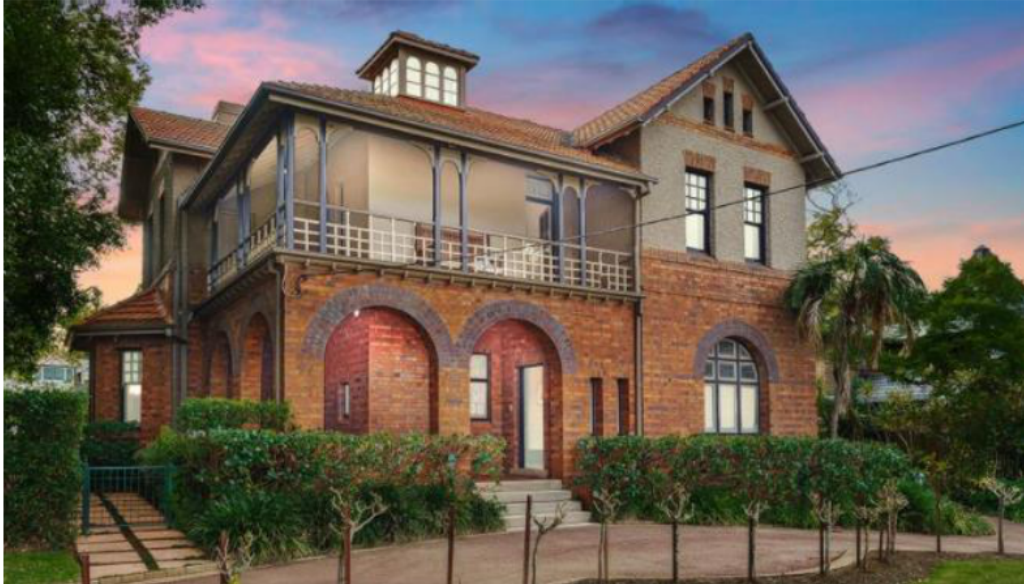
Figure 16: Primary elevation (south) from Ethel Street (Source: realestate.com.au, accessed September 2020).
