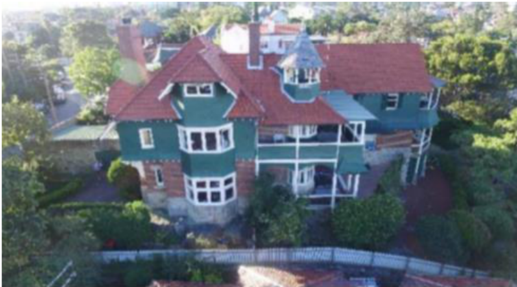
Figure 77: View showing the southern elevation of Hollowforth. Note: the Belvedere/belfry tower and timber shingles periodically fall.
