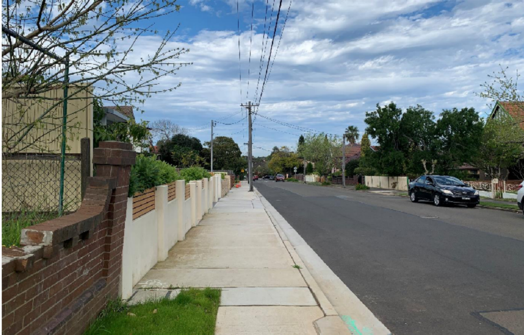
Figure 9: View east from 11A Ethel Street.
