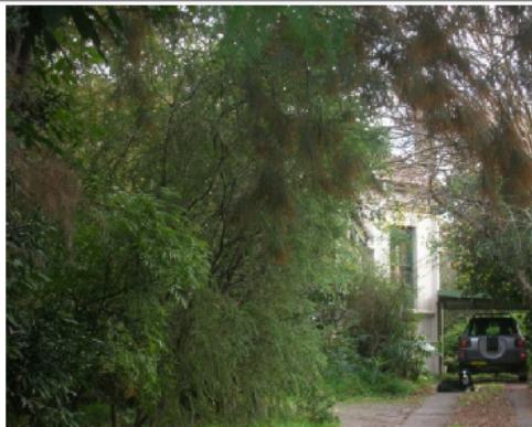
Figure 65: View to the house from Lindsay Street (Source: State Heritage Inventory Form for 'Victorian House [Item 69]', database no. 1250176, accessed November 2020).
