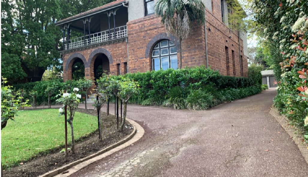
Figure 18: View toward the primary (southern) and eastern elevations and gravel drive leading to the garage at the rear of the site. Note: the plantings to either side of the turning circle and drive, and exposed facebrick to both ground and first floors of the eastern elevation.
