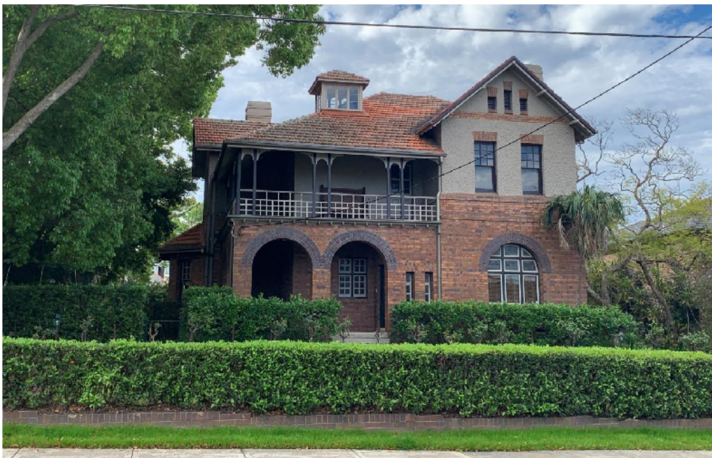
Figure 15: View north from Ethel Street to the primary façade of the main building within the subject site. Note: the facebrick ground floor and roughcast rendered upper storey, verandas, tiled terracotta roof, painted brick tall chimney and central belvedere/belfry.
