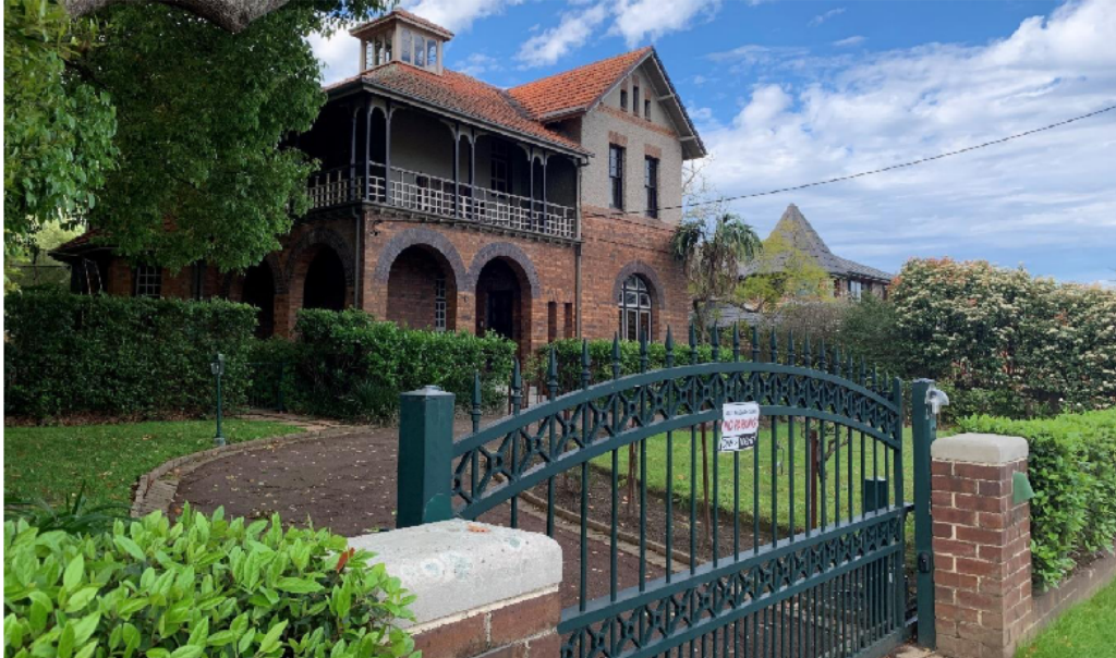
Figure 14: View north-east from Ethel Street towards the subject site showing the front garden, hedge and brick fencing, cast iron entry gate (west), gravel turning circle and primary façade to the main house.
