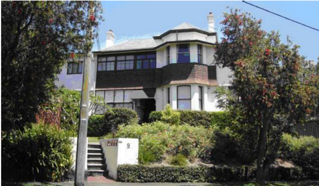
Figure 67: Primary façade to Dunbrody from Davidson Parade (Source: State Heritage Inventory Form for 'Dunbrody', database no. 2181075, accessed November 2020).
