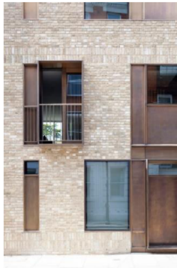
Recessed openings add depth to the overall façade. (Source: GMU Library)
