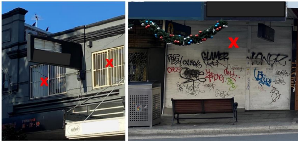
Figure 1(g). Examples of prohibited security bars, shutters or permanent grilles and air handling systems.
