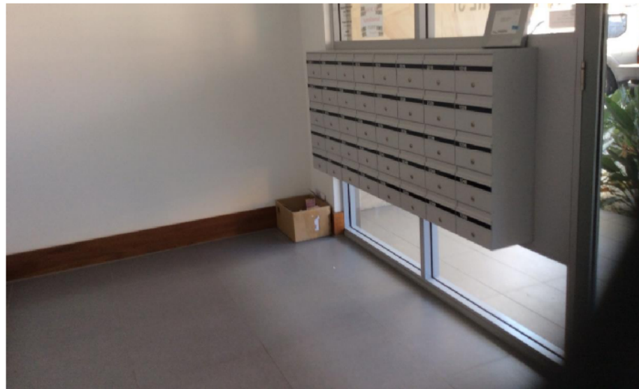
Figure 1(b): Example of Mailboxes Accessible from a Secure Internal Foyer
