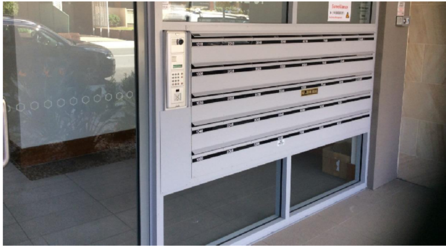
Figure 1(a): Example of Mailboxes Integrated into the Front Wall of a Residential Flat Building
