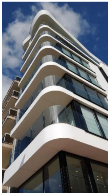
Changing the façade material, articulation or colour to highlight prominent corners. (Source: ADG, 4M)
