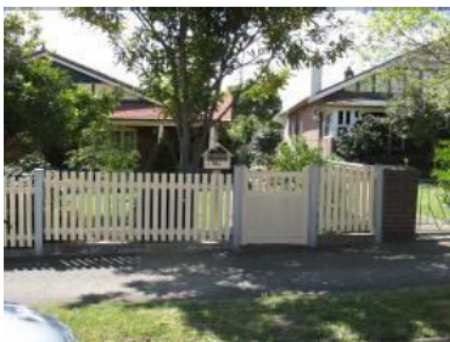
Inter-War Bungalow Timber Paling Fence and Gate
