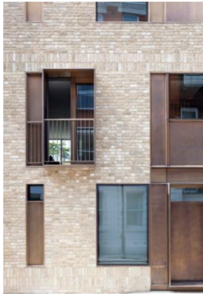
Recessed openings add depth to the overall façade. (Source: GMU Library)
