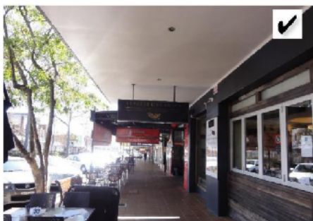
Under awning supporting structures, wiring and lighting should be concealed unless they are consistent with the character of the building.
