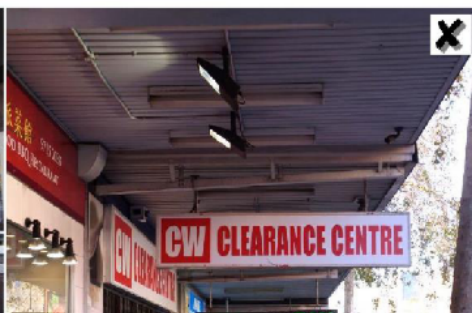
Exposed lights are not encouraged unless they are fitted and integrated within the fascia or consistent with the character of the building.
