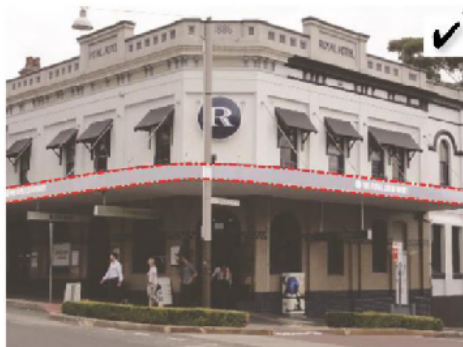
Continuous splayed awning around the corner
