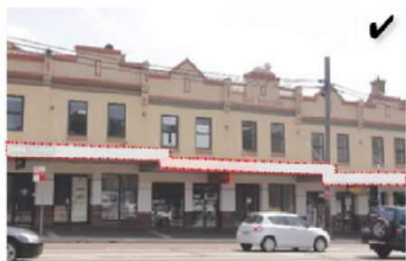
Awnings are to step down to follow the terrain/level of the street.
