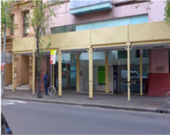
Example 11: Gantry Style – Acceptable in all zones
