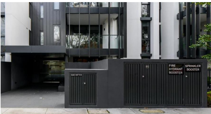
Examples of good sprinkler booster and fire hydrant enclosures.
