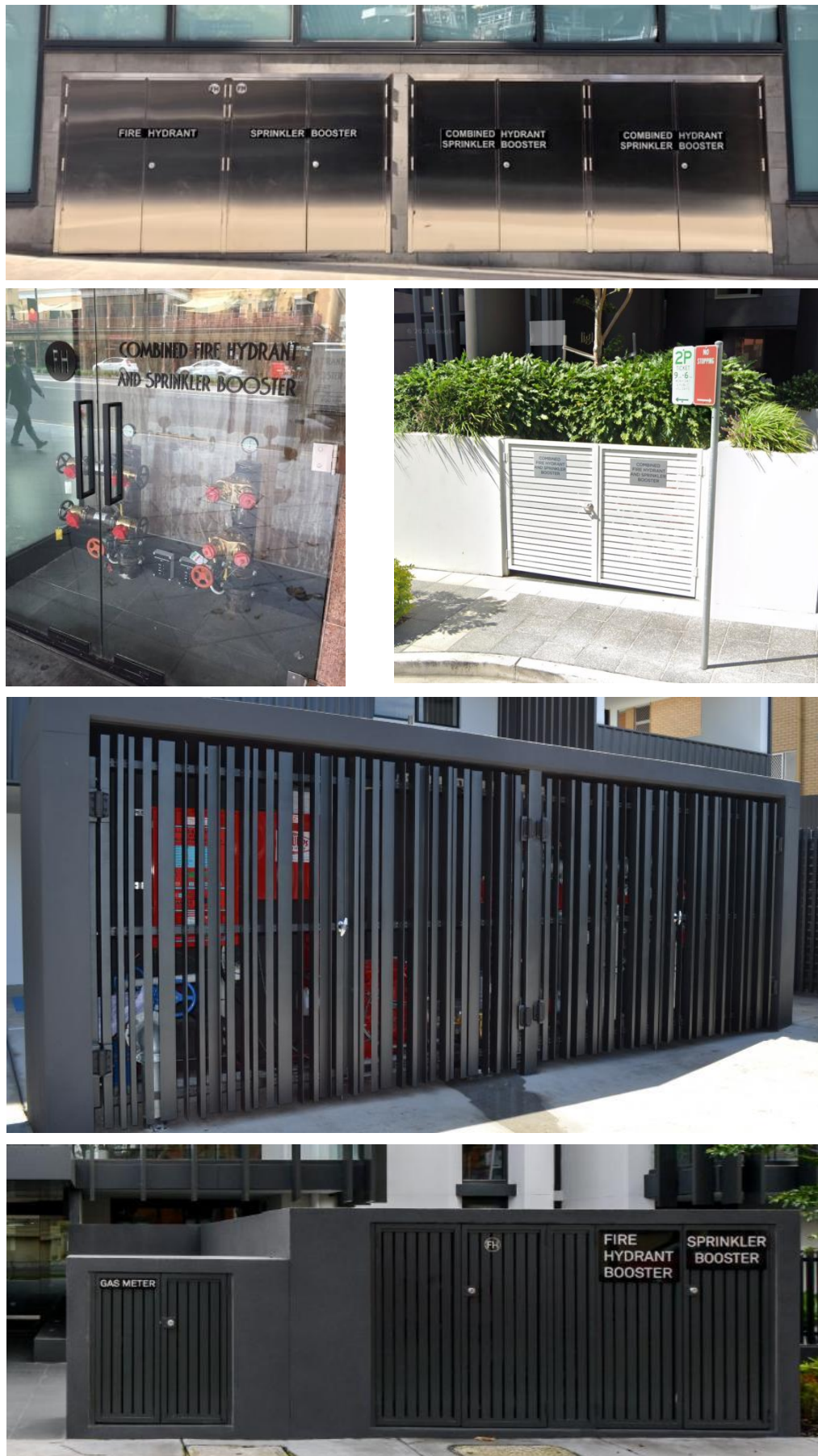
Figure 1(c) Examples of enclosed fire safety utilities
