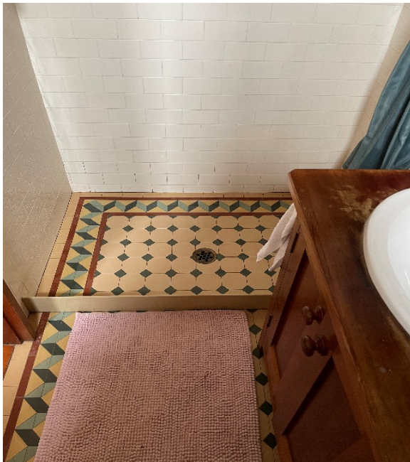
Figure 4.25 The floor of the non-original bathroom in the rear extension incorporates traditional tiling pattern.
