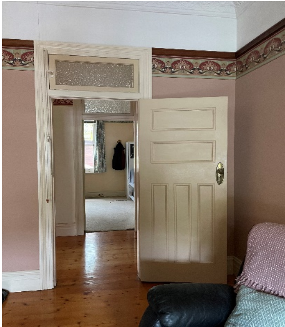
Figure 4.19 View of an original internal door with intact hardware details.
