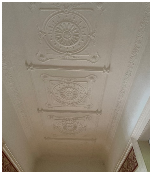
Figure 4.10 The decorative plaster ceiling along the central hallway.
