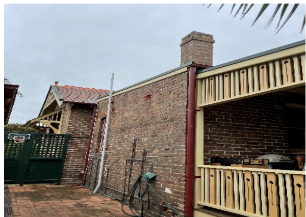
Figure 4.6 The eastern façade of the dwelling showing the original brick chimney.
