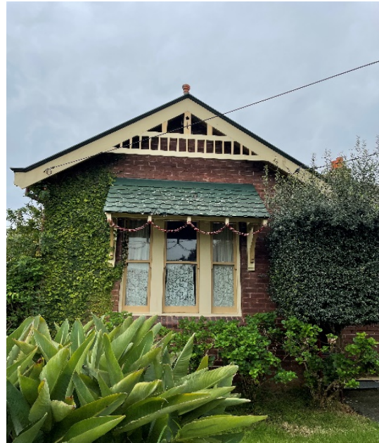
Figure 4.8 The projecting bay along the features an ornate gable end and timber-framed double-hung casement windows with a slated awning.
