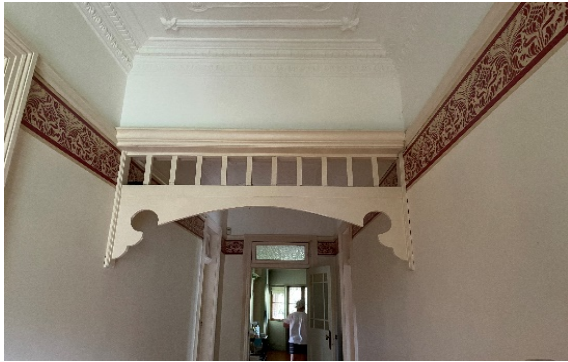
Figure 4.11 The timber fretwork arch along the central hallway.
