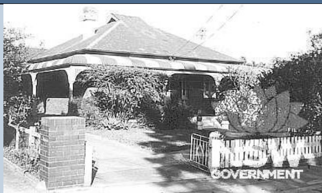
Figure 5.2 1986 photograph of 8 Seale Street. (Source: Fox & Associates Architects/Planners Sydney, sourced from the State Heritage Inventory)
