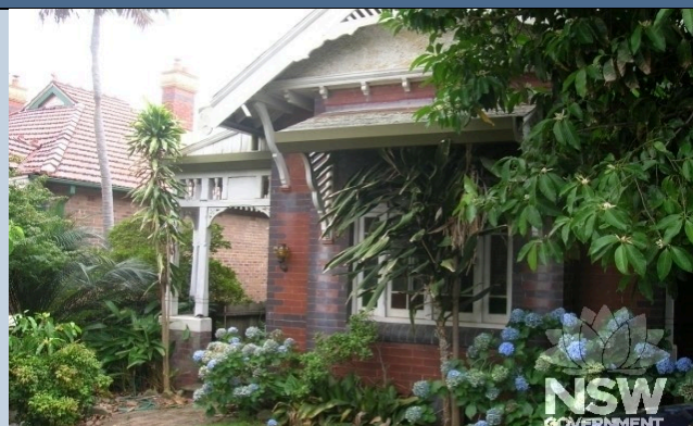
Figure 5.4 View of the projecting bay with a gable end along the primary façade. (Source: State Heritage Inventory)
