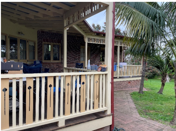
Figure 4.5 View to the non-original verandah along the rear façade of the dwelling.
