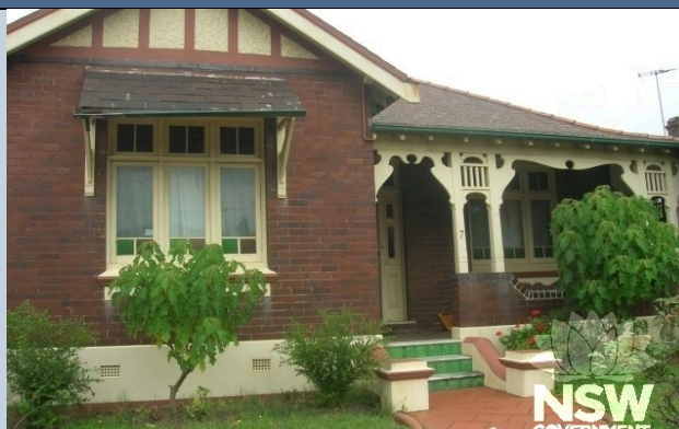
Figure 5.6 View of the projecting bay and the front verandah along the primary façade. (Source: State Heritage Inventory)
