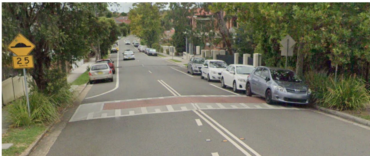
Concrete Raised Threshold
