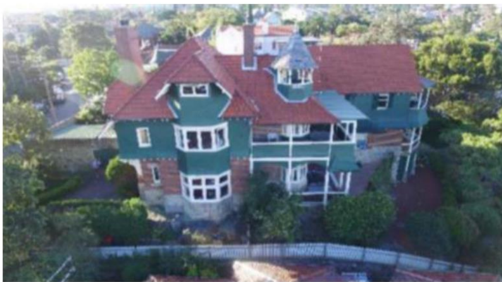
Figure 77: View showing the southern elevation of Hollowforth. Note: the Belvedere/belfry tower and timber shingles periodically fall.
