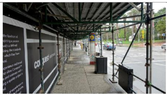
Example 14: Underside of hoarding must be painted white
