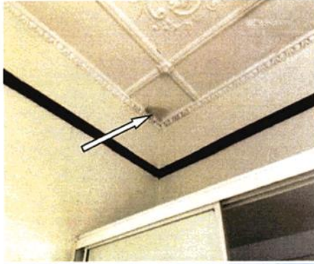
DAMAGE ON THE CEILING LINING
