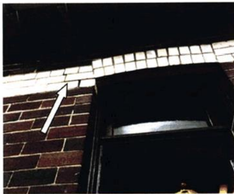
FACE BRICKWALL CRACK ABOVE WINDOW OR DOOR
