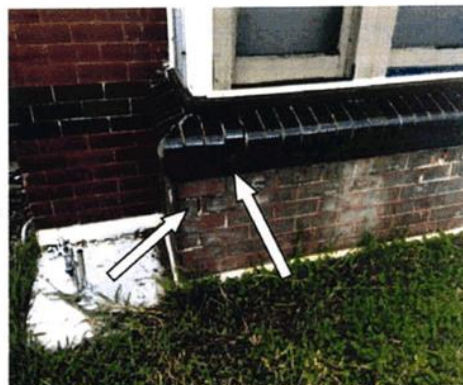
WINDOW SILLS DISLODGED AND BRICKWALL CRACK
