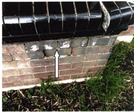
FACE BRICKWALL CRACK BELOW WINDOW SILL
