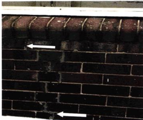
FACE BRICKWALL CRACK BELOW WINDOW SILL
