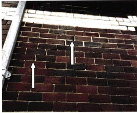
FACE BRICKWALL DIAGONAL CRACKING
