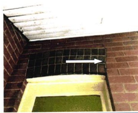
FACE BRICKWALL CRACK ABOVE WINDOW OR DOOR
