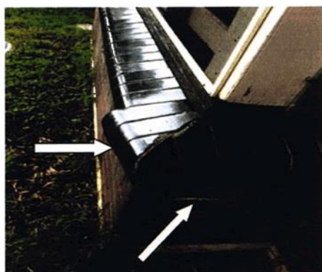
WINDOW SILLS DISLODGED AND BRICKWALL CRACK
