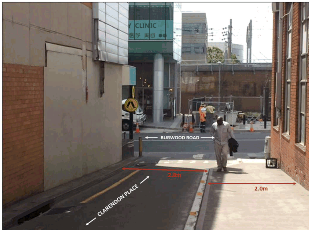
Completed Footpath Widening
