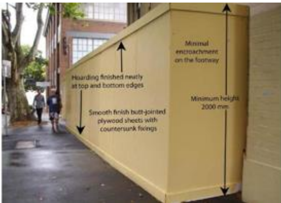
Example 5: Painted - Acceptable in Commercial Zones
