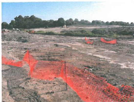
Plate 3: Site looking North-East
