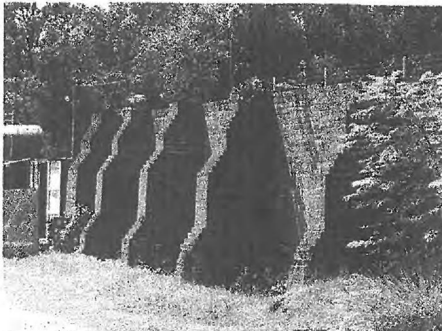
Photograph 3: the western section of the brick retaining wall
