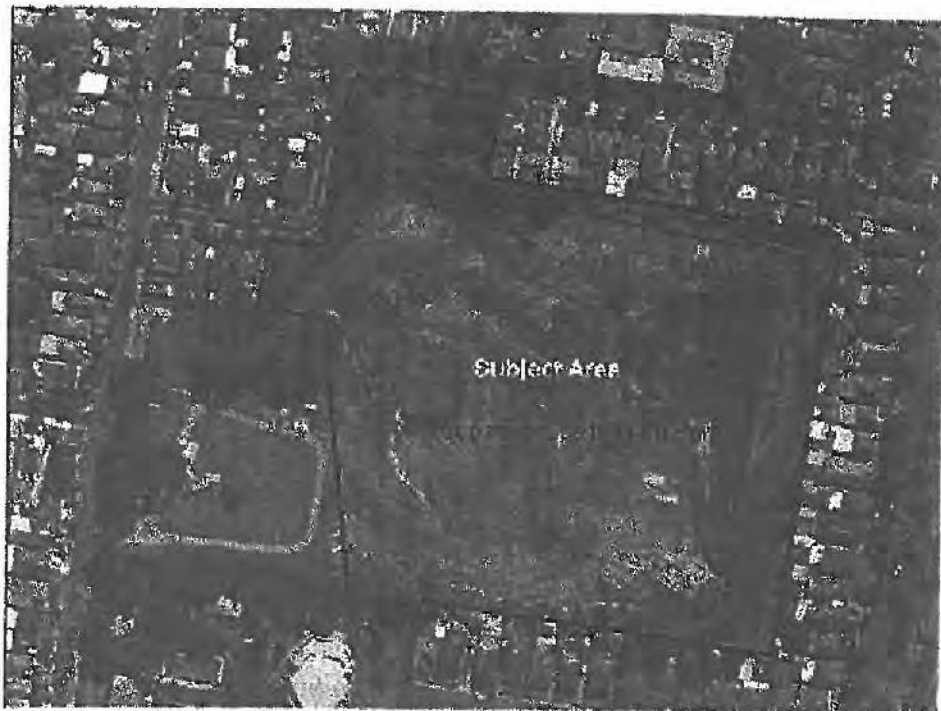
Figure 7: Aerial photograph of the site taken before some of the remaining structures were removed. Reproduced courtesy of Burwood Council
