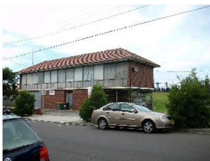
Figure 23 - SES building on Cheltenham Road
