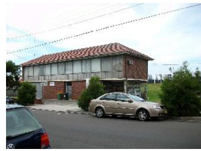
Figure 10 - State Emergency Services Headquarters (March 2013)
