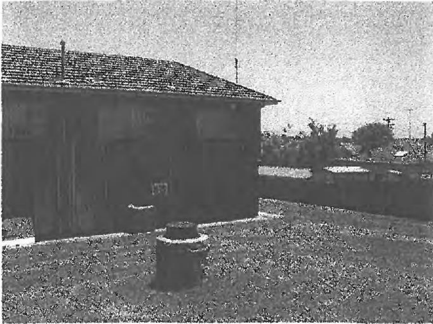
Photograph 6: remnant chimney at the rear of the former Brickworks Limited head office in the subdivided section of the former site
