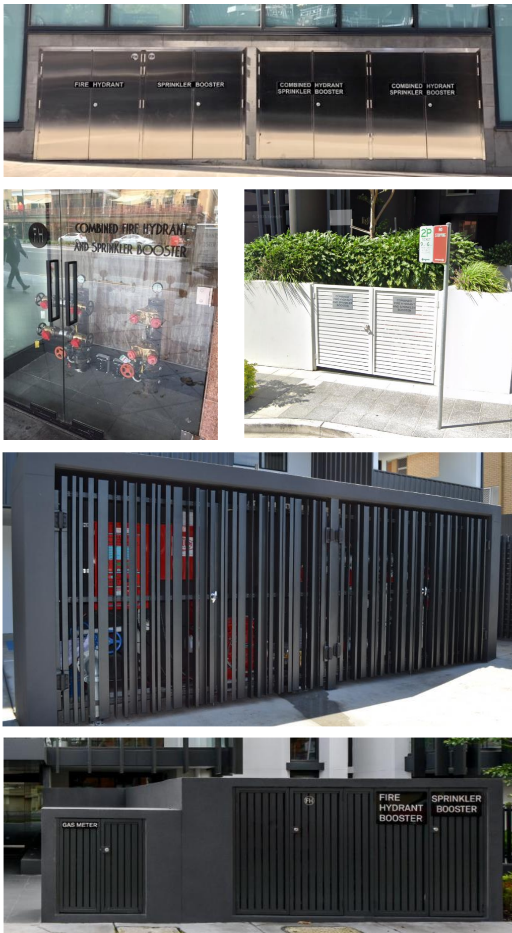
Figure 3. Examples of enclosed fire safety utilities
