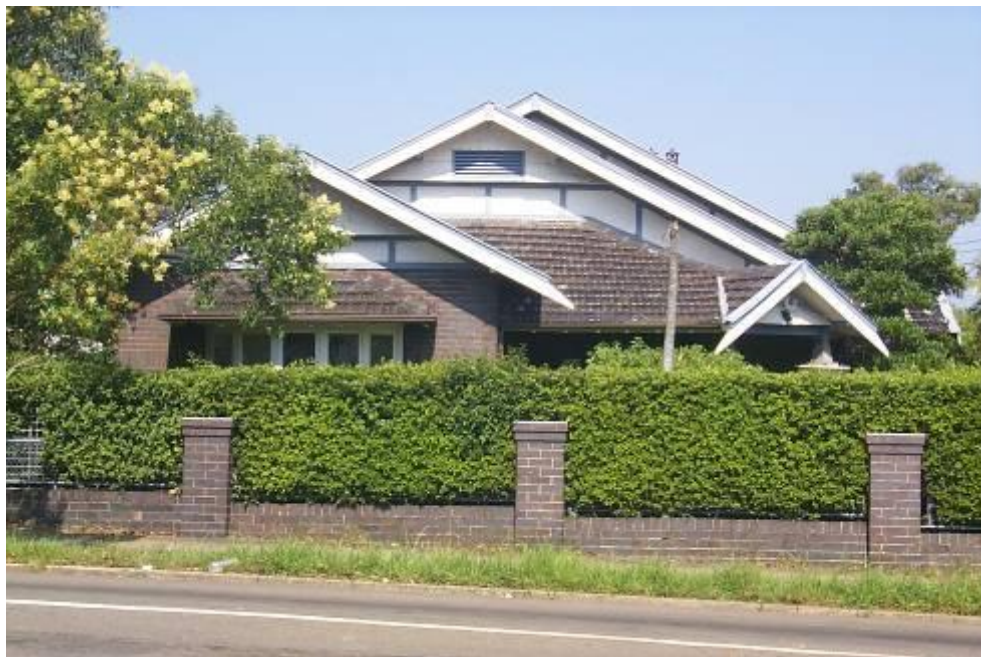
Figure 87. Asymmetrical roof forms
