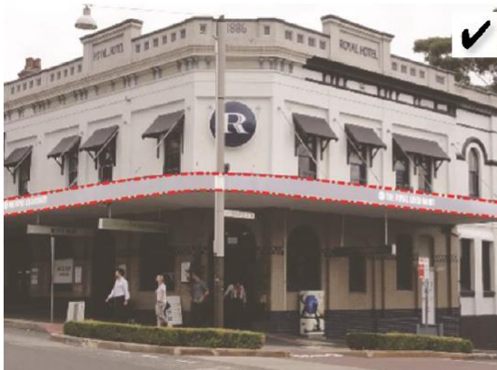
Continuous splayed awning around the corner
