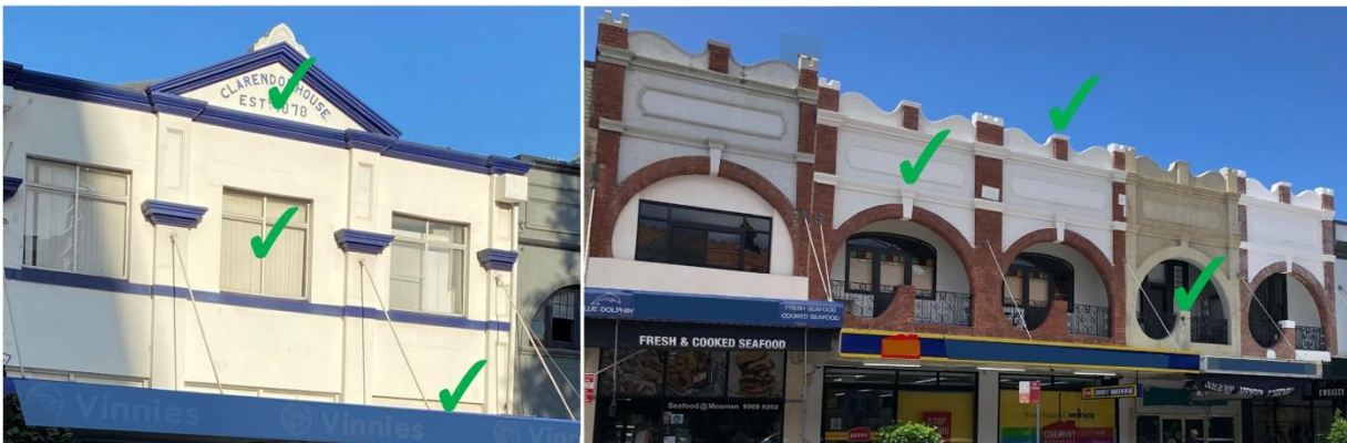
Figure 8. Examples of good quality facades without security bars, permanent grilles or air handling systems
