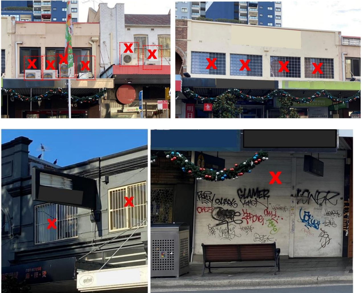
Figure 7. Examples of prohibited security bars, shutters or permanent grilles and air handling systems
