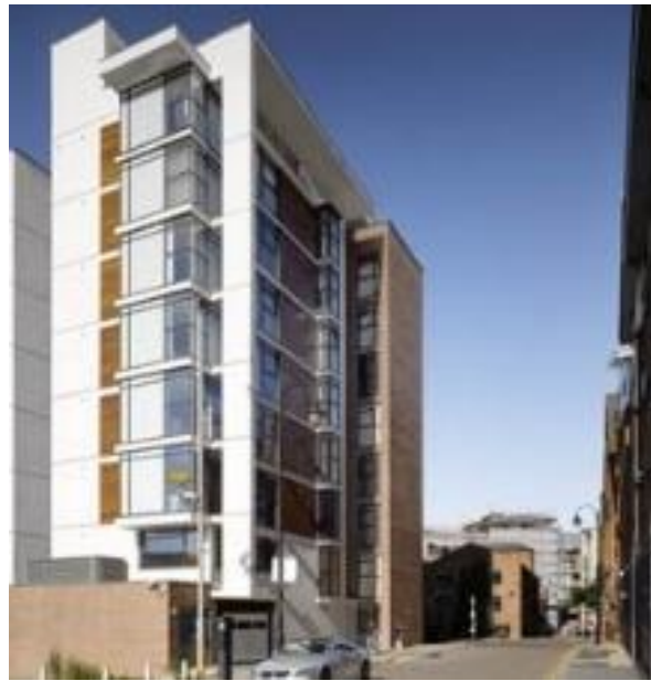
Primary materials are associated with the majority of the elevations of the building. (Source: Auckland Design Manual)
