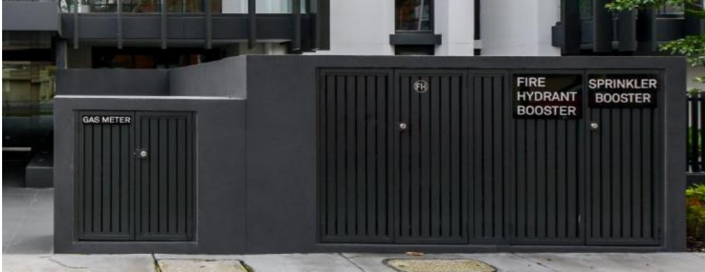
Figure 3. Examples of enclosed fire safety utilities
