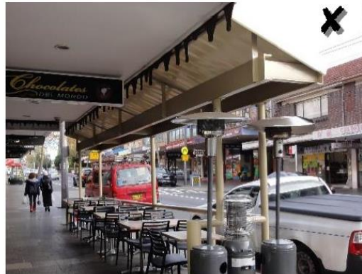
Permanent awning extension structures can obstruct visual connections between both sides of the street.
