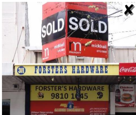
Signs with multiple contrasting colours, text not proportional to the building and permanent above awning signs are not permitted.
