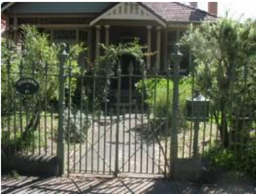
Victorian Cast Iron Pickets and Gate
