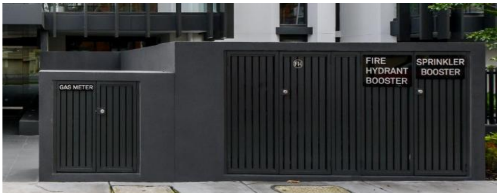
Figure 1(c) Examples of enclosed fire safety utilities
