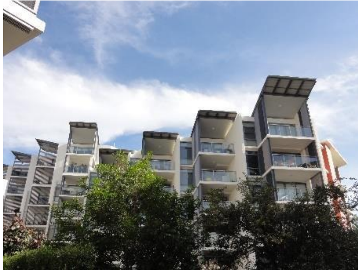
Examples of the roof character integrated with the overall façade design. (Source: GMU Library, Google)
