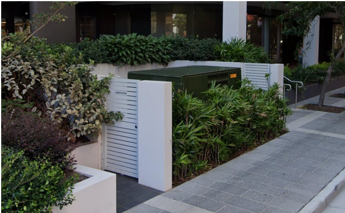
Figure 1(d): Example of a screened large power supply utility / substation
